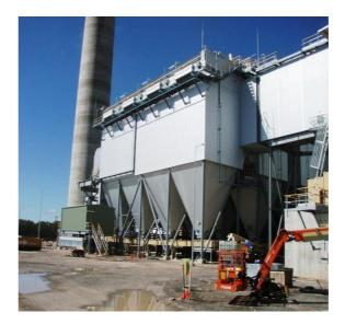
Alstom fume treatment centres with AHEX deliver improvements in smelter energy balances whilst reducing gas cleaning footprints. This makes them flexible alternatives to conventional conditioning towers and dry scrubber reactors.
